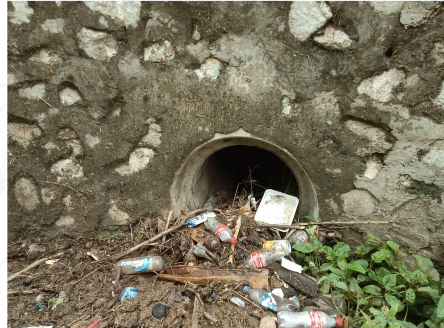
Blockage of drainage with household wastes and debris
